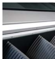
Continuous skirt panel lighting 1
